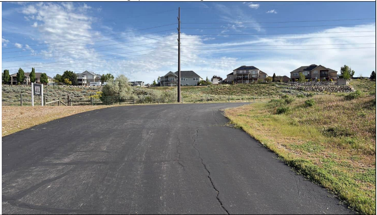
Photograph 6. View Looking North from Point D
